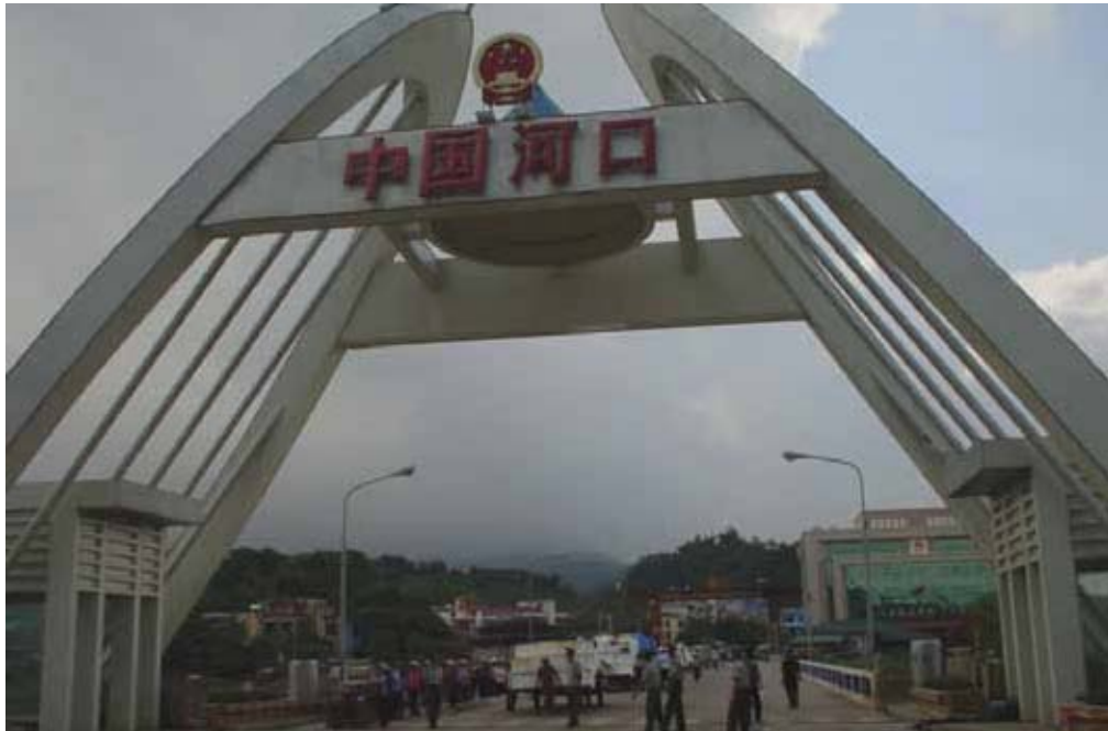
Bridge linking the Hekou (PRC)—Lao Cai (Viet Nam) border crossing.
